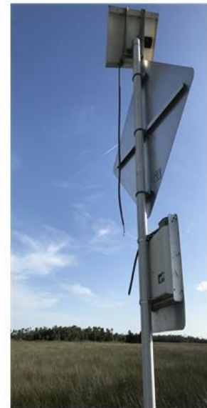
Broken cable at Site 16 (EB, 28°50'07.8"N 82°37'24.6"W)
